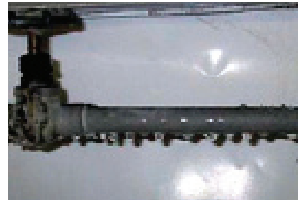
Moisture condensing on the outside of compressed air pipework (sweating)
