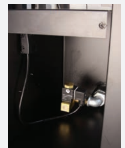
SmartDrainer - Drain valve
