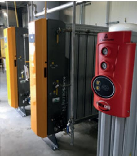
2 x N2-55P nitrogen generators and an MXS102c desiccant dryer pre-treatment package provide food grade nitrogen at 0.5% purity to Taylor Farms for MAP.
