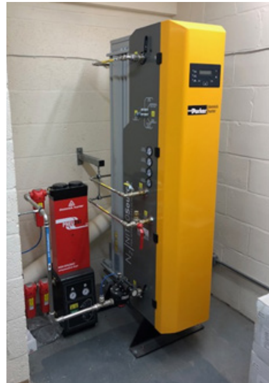
N2-20P for twin pot soldering machine. Installed nicely in small space to side of factory.
