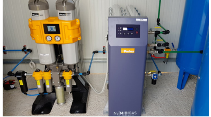
MIDIGAS6 and CDAS installed using Transair by ITO at Saint Dimitrios Cooperative
