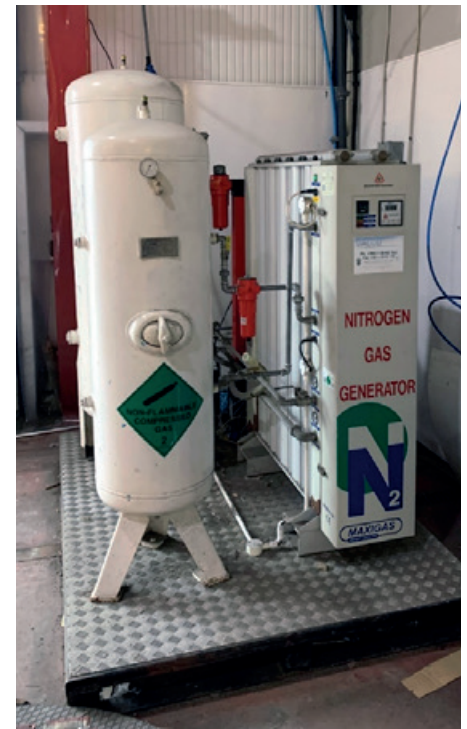
Existing N2MAX110 skid - 20 years old!
